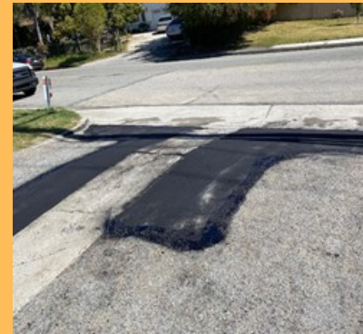
Road Repair Work on Mountain Avenue (Ward 4)
